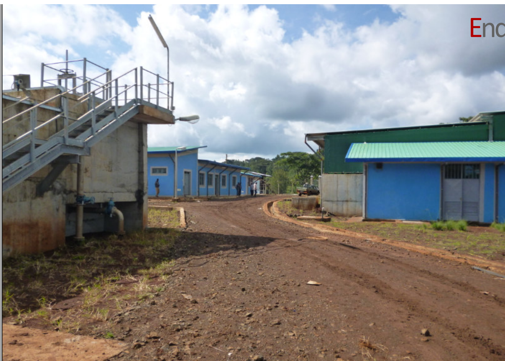
Dembidollo Water Treatment Plant Ethiopia
