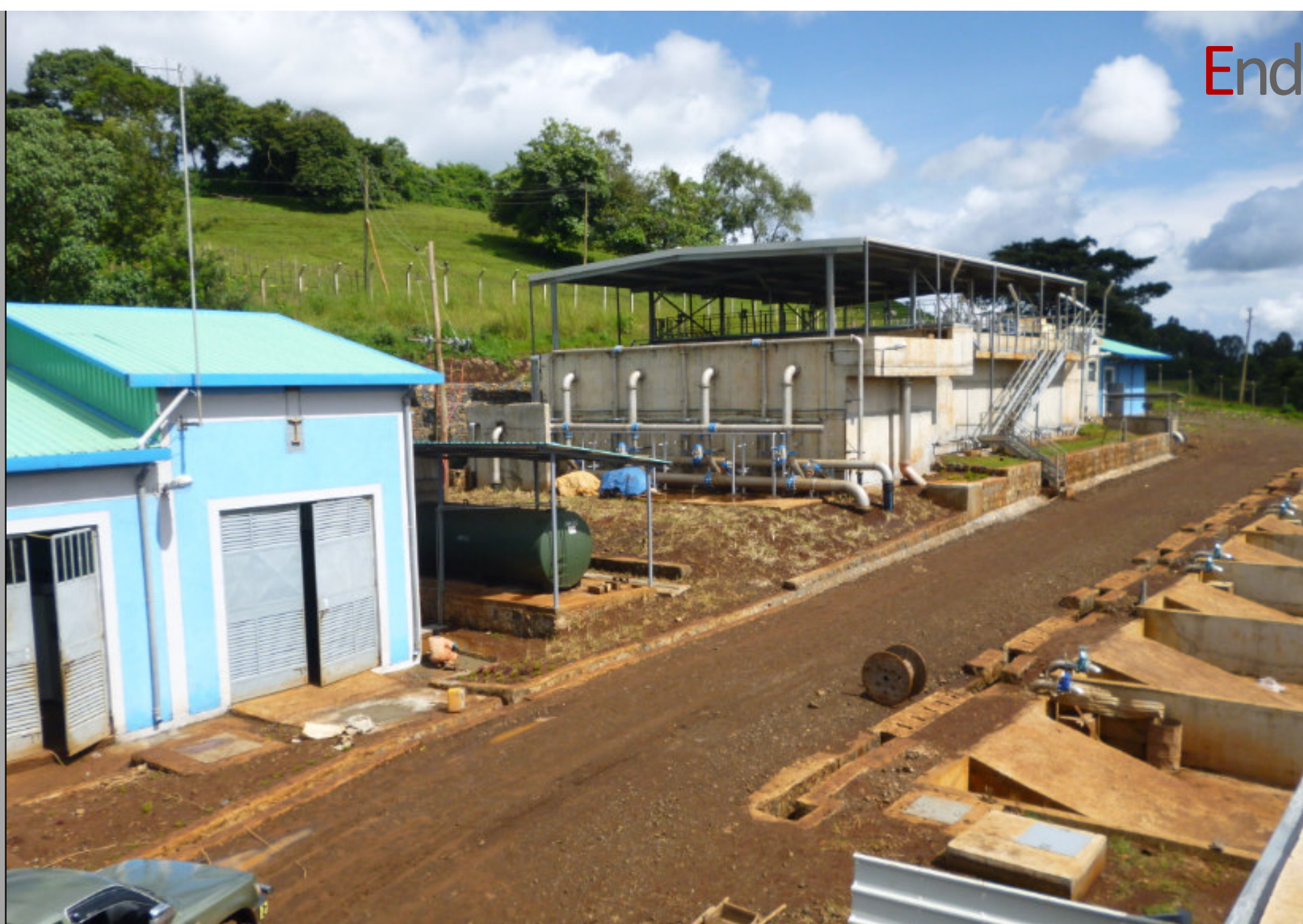
Dembidollo Water Treatment Plant Ethiopia
