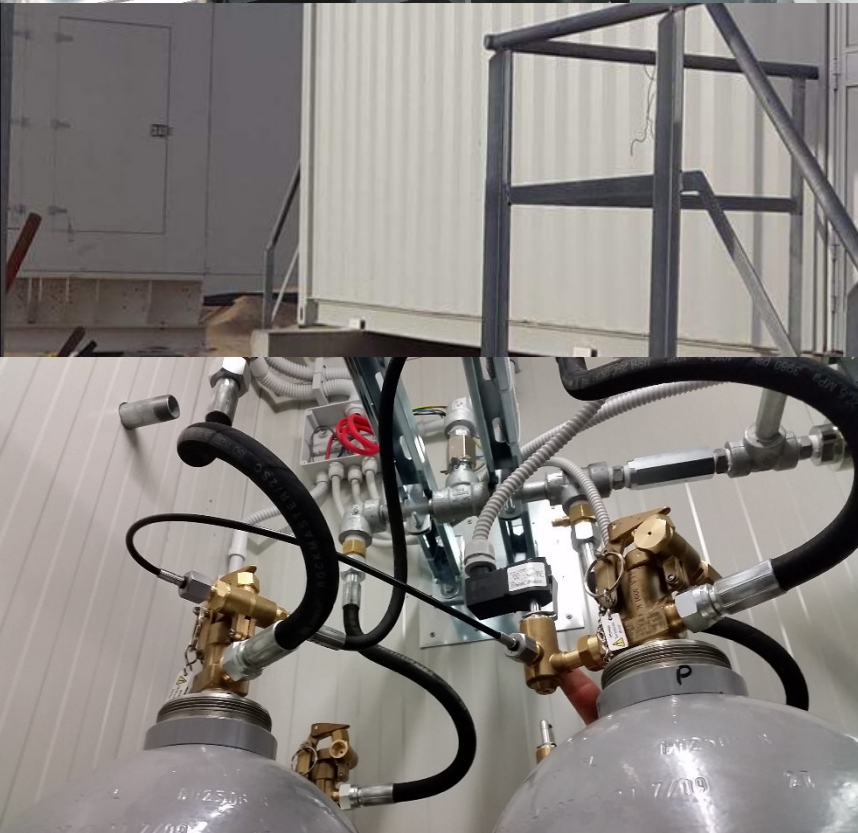
Electrical BOP for Solar MPU
