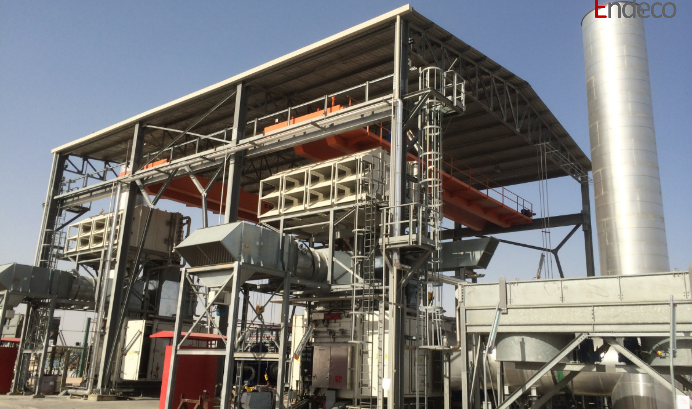
Tuba Turbogas Oil Pumping Station
